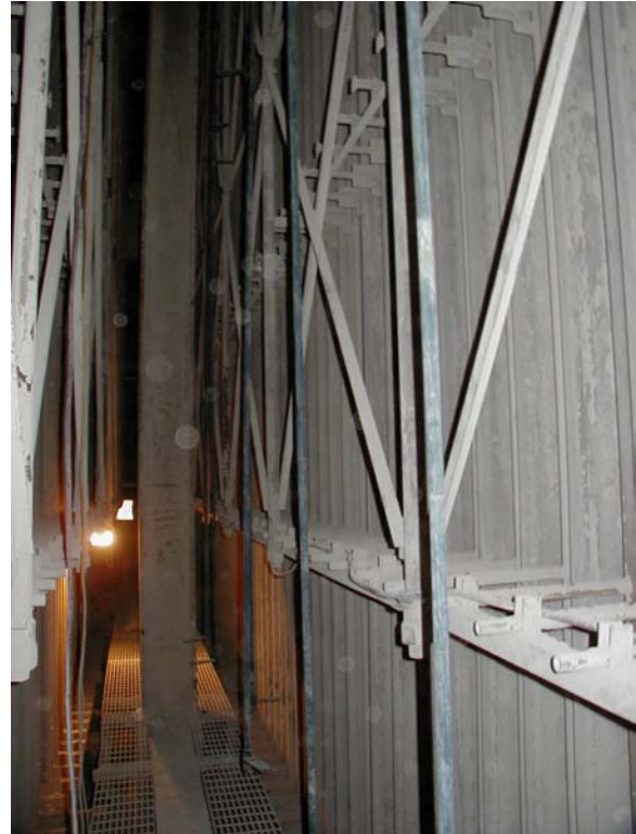
Figure 5. Injection Grid Between ESP Fields.
